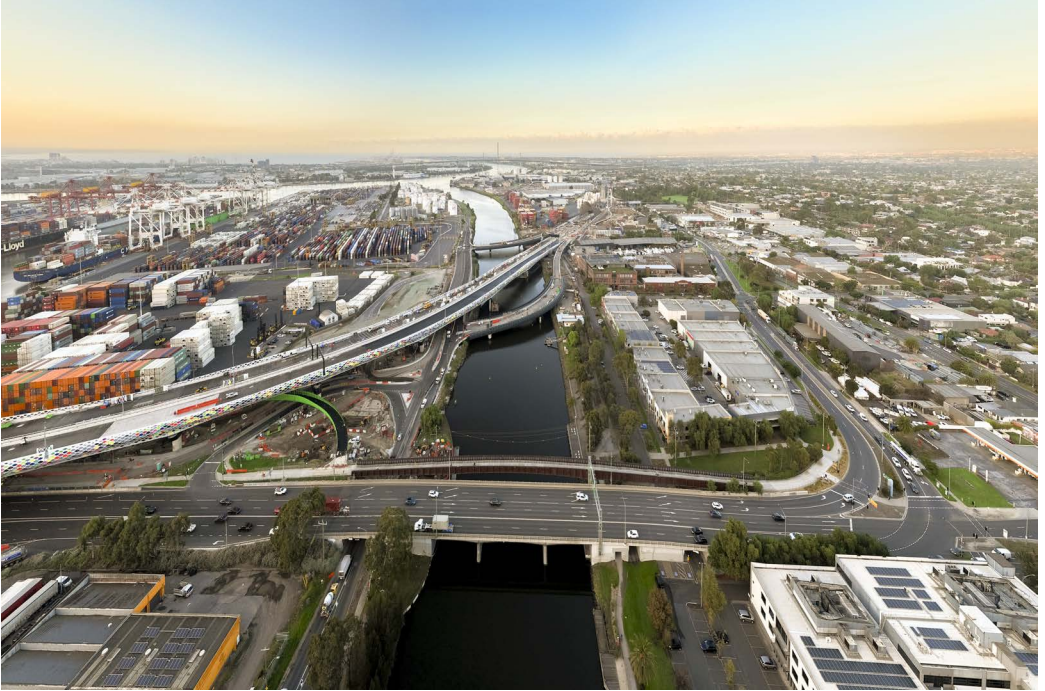
The new Maribyrnong River crossings and West Gate Tunnel entrance near Port of Melbourne, March 2025. Photo courtesy of Port of Melbourne.
