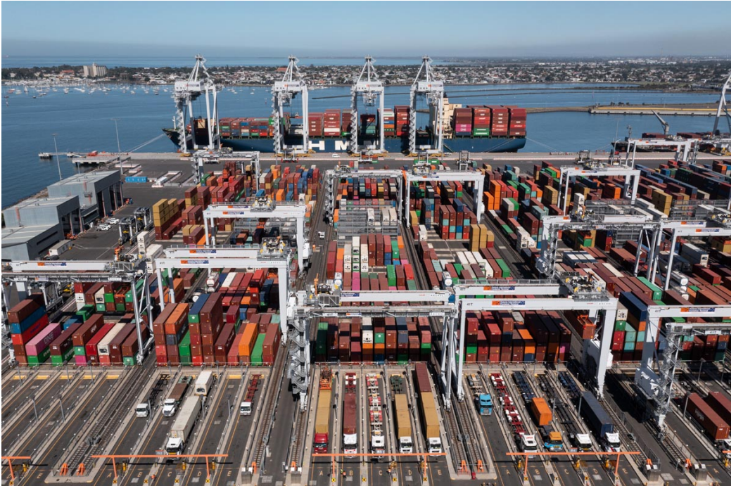
Container operations at Victoria International Container Terminal (VICT). Automated stacking cranes (ASCs) receive and deliver containers to the landside, while remotely-operated cranes load a vessel at berth. Photo courtesy of Port of Melbourne.
