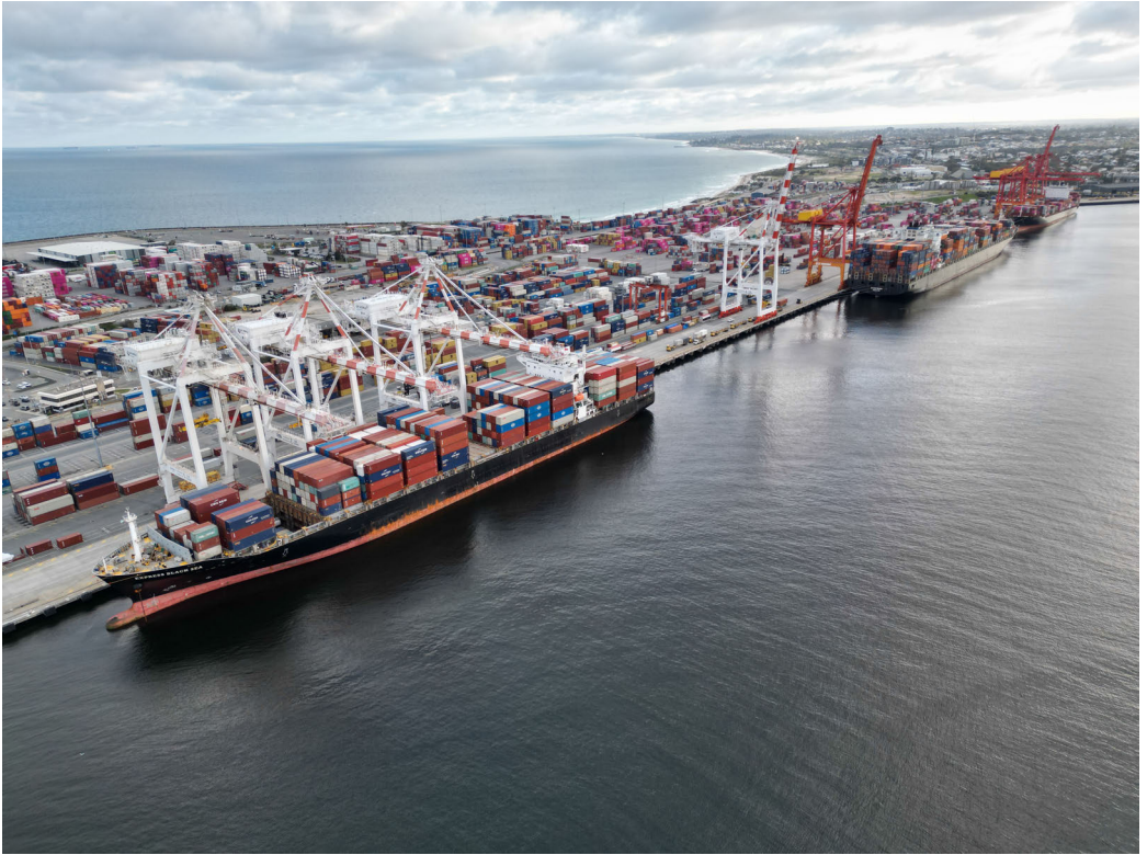
Aerial view of the North Quay container berths at Fremantle Inner Harbour, September 2024. Photo courtesy of Fremantle Ports.
